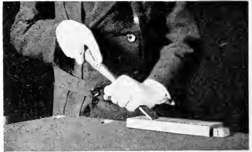
Fig. 22. Whetting the Beveled Side of a Chisel.
